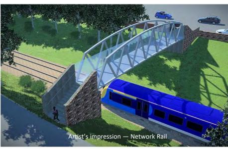
The selected design for Network Rail's new footbridge at Strathbungo Scotland. The infill of all of the 'V' shaped struts is of a toughened clear material to maintain an open look to the bridge.
